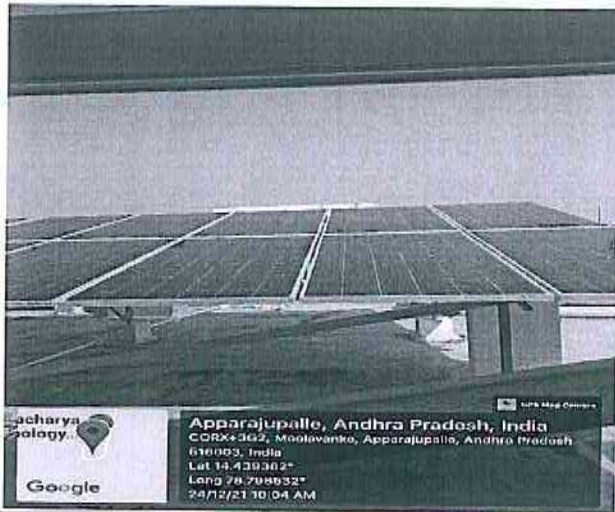
Rooftop Grid Connected Solar Power Plant (100 kWp)
